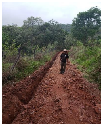
Pipe line for the water system
